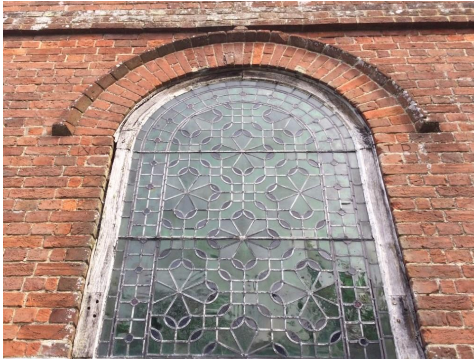
Fig 1. West wall window with initials WC and TD to either side of window. Photo KP12
