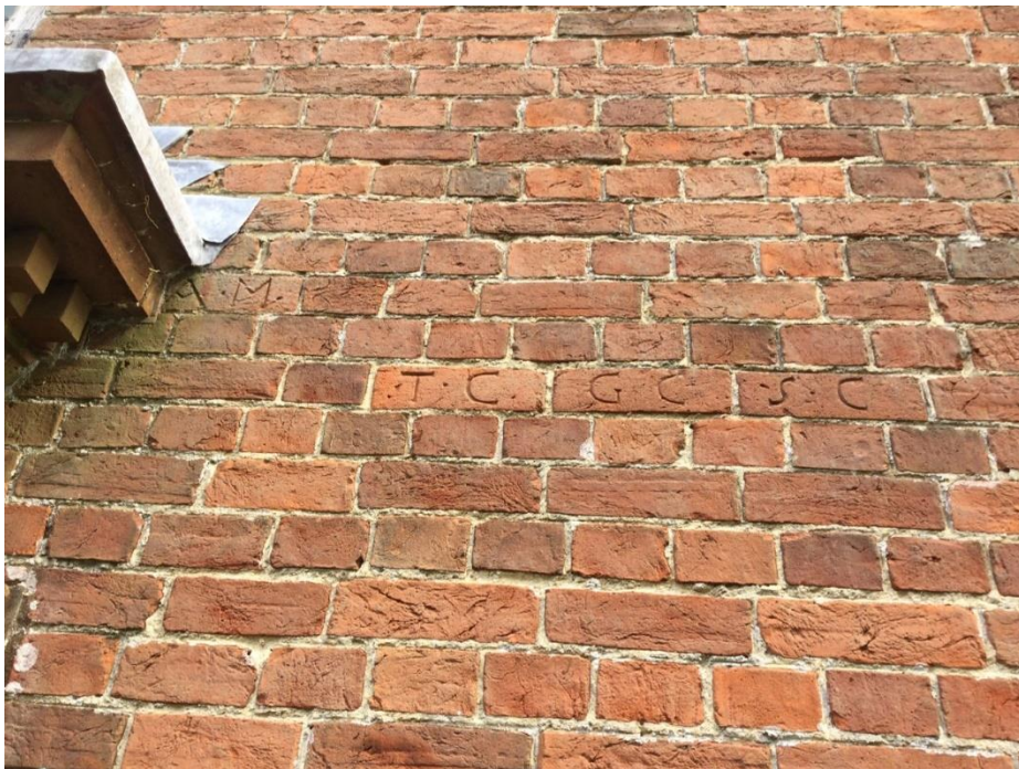
Fig 2. Exterior west wall. Initials T.C, G.C, S.C, A.M. Photo KP10
