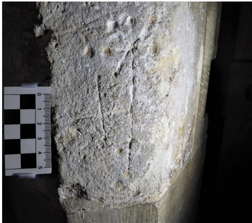
Fig 18. Chancel doorway within vestry porch east side. Crosses. Photo KW4.
