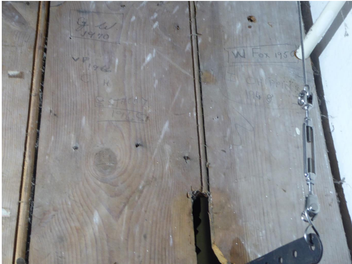
Fig 21 Bell ringing chamber clock cupboard. Initials, names and dates. Photo KW27
