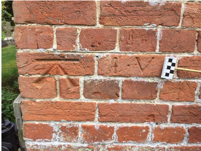
Fig 3. External west wall. Cut mark benchmark and initials I.V. Photo KP13
