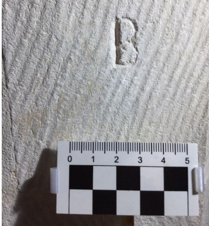
Fig 17. Sanctuary window ledge. Initial B. Photo KP61
